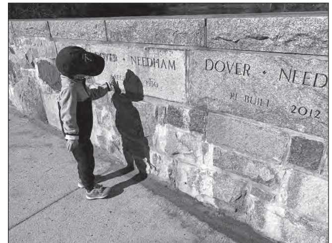
Dover-Needham Bridge. Photo by Carol Lisbon.
